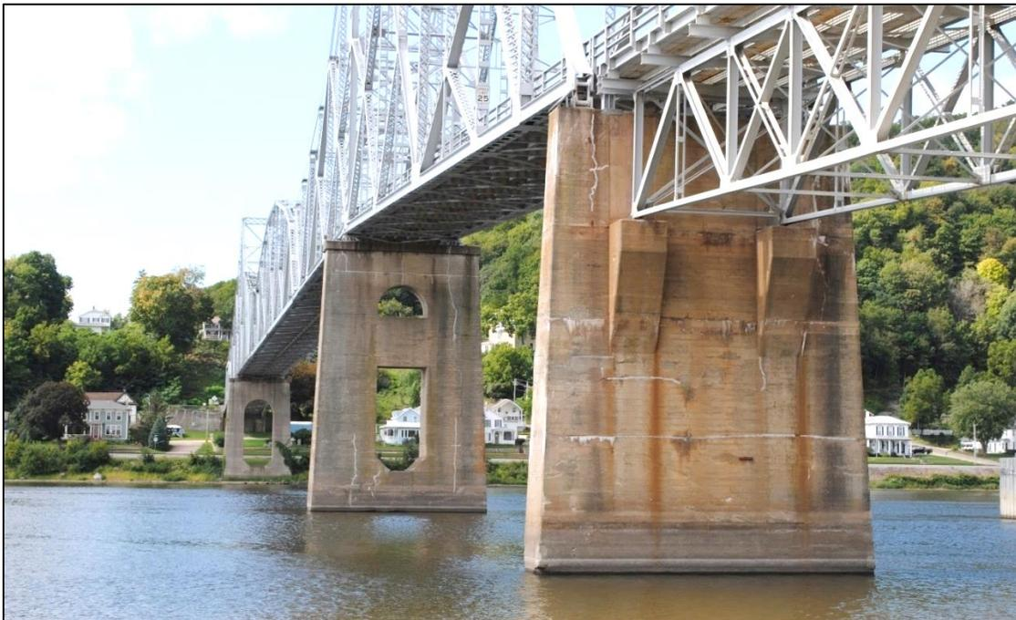
**Figure 18. Piers 1 through 3 as seen from Wisconsin, looking west. Note the two concrete truss supports on the east elevation of Pier 3 and the differences in design of the openings on Pier 1 and Pier 2. Source: Tallgrass Archaeology LLC, September 18, 2022.**
