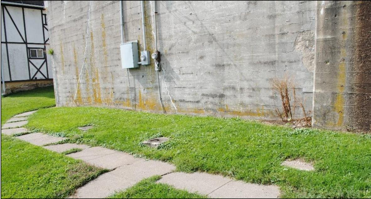
**Figure 22. Three concrete pads between the sidewalk and concrete abutment. These once held posts that upheld the overhanging building on the upper level. Electrical/switch boxes are also seen affixed to the abutment, looking southwest. Source: Tallgrass Archaeology LLC, September 18, 2022.**
