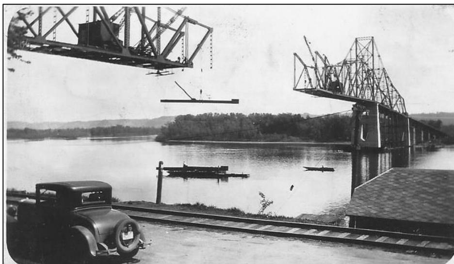
**Figure 37. Construction of superstructure over the main channel, looking northeast.**
