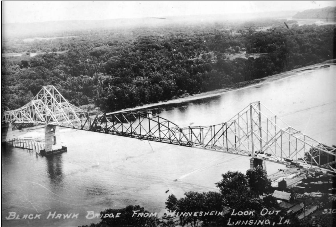
**Figure 40. Circa-1931 photograph showing coffer dam components around the second and third piers still in place at or near the time the bridge was completed, looking southeast from bluff.**
