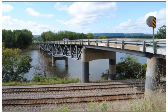
Figure 26. 1956 deck truss bridge over Winneshiek Slough and railroad, east end abutment at WI-35, looking northwest. Source: Tallgrass Archaeology LLC, September 18, 2022.
