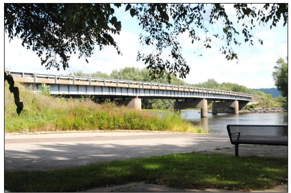
Figure 27. West 1956 slough bridge, at Big Slough Boat Landing, looking northeast, an example of concrete and steel girder slough bridge design. Source: Tallgrass Archaeology LLC, September 18, 2022.
