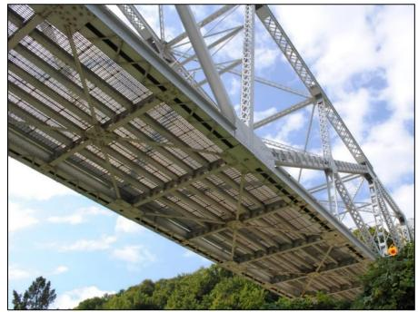
Figure 16. View from below of steel grid deck and braces across bottom of the bridge, looking southwest under the west span. Note the visibility through the deck. Source: Tallgrass Archaeology LLC, September 18, 2022
