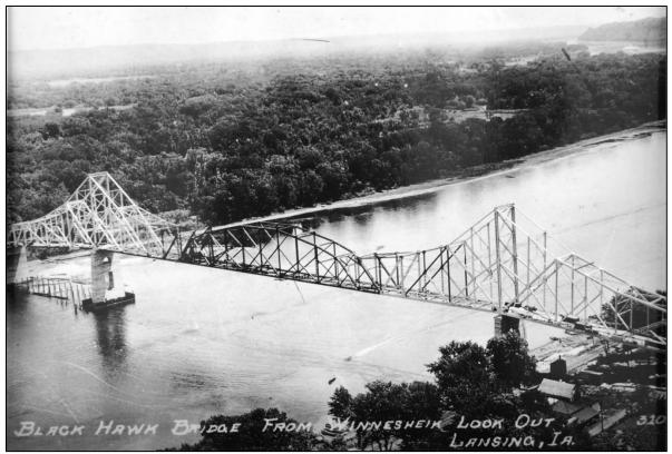
Figure 40. Circa-1931 photograph showing coffer dam components around the second and third piers still in place at or near the time the bridge was completed, looking southeast from bluff. Source: Private collection of Sam & Betty Bell, 2022.
