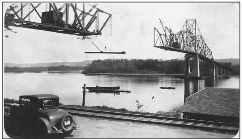
Figure 37. Construction of superstructure over the main channel, looking northeast. Source: John Rethwisch private collection.
