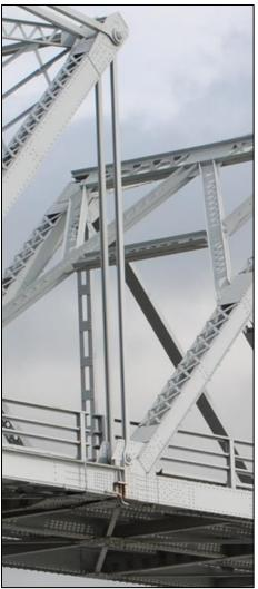
Figure 10. Detail view of suspension-cantilever connections including pin connection, looking northeast. Source: Tallgrass Archaeology LLC, September 18, 2022.
